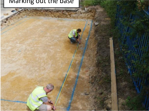
Marking out the base
