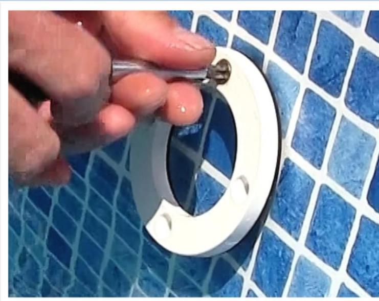
Undo the top screw and insert it back through the face plate, into the same hole it came from. Give the screw a couple of turns just to hold on to the face plate. When the face plate swings downward you can locate the bottom screw and carry out the same procedure.
