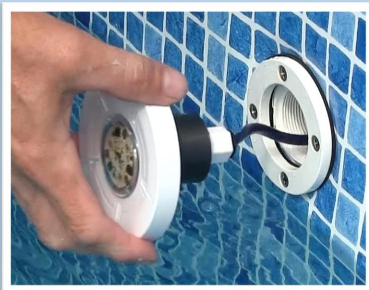
Now the light fitting in the pool wall is exposed, you need to get the cable from the light up through the conduit into the deck box. where a connection can be made.
