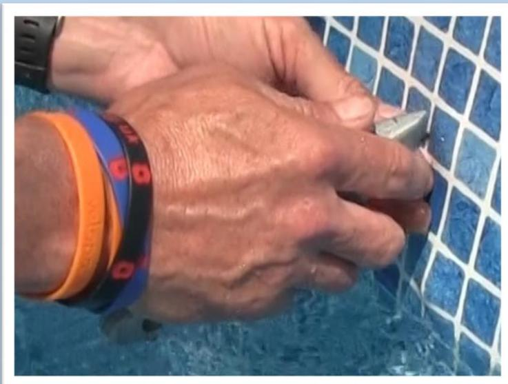
On the inside of the pool allow the water level to rise just below the light fitting which is now behind the liner. Carefully feel for the screws.
