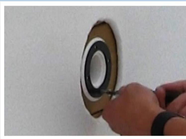
Insert a screw top and bottom, do not fully tighten the screw and finish with the cross of the screws pointing North, East, South and West.
