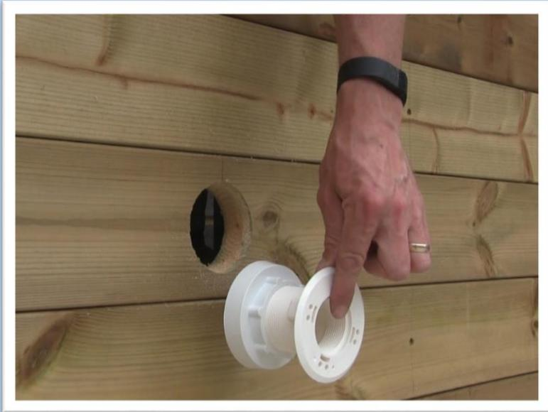
The fitting used as shown, uses a back nut in this sequence (shown), to tighten against the pool wall.
