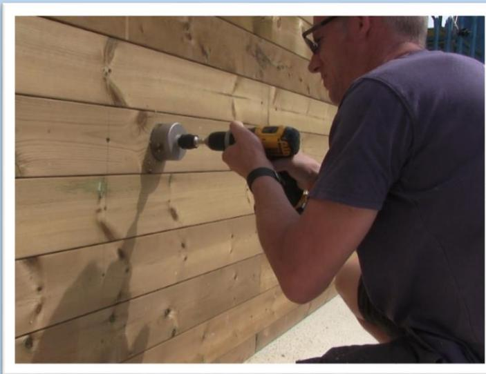
Use an 85mm hole cutter to cut the hole for the light. Do not drill through the wall in one go. from one side.
