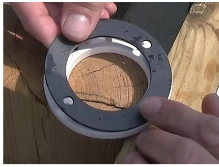
Line up the holes and stick the gasket to the face plate.
