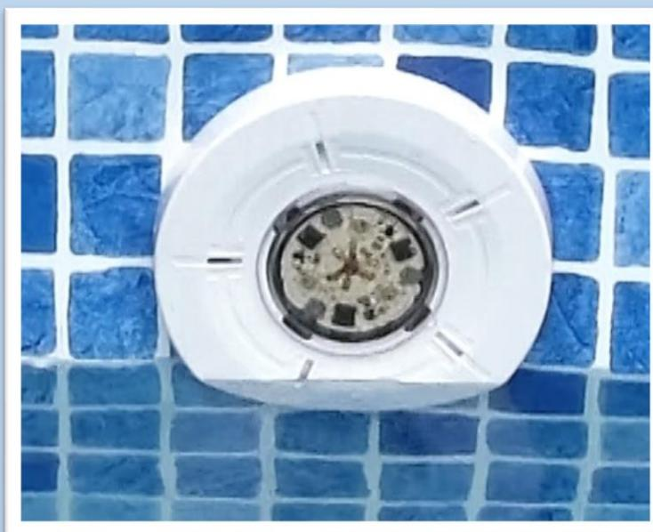
Once you have secured the cable in the deck box you can screw the light fitting in place.
