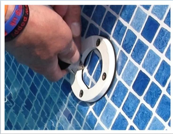
You can now insert the other two screws and tighten all four screws using a hand-held screwdriver.
