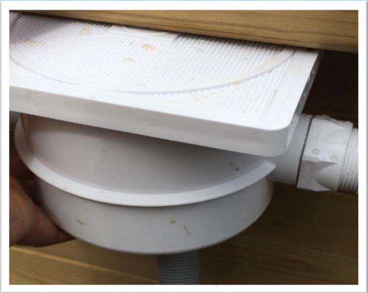
With the other end of the conduit apply plenty of PTFE tape to the thread and screw it into the bottom of the deck box.
