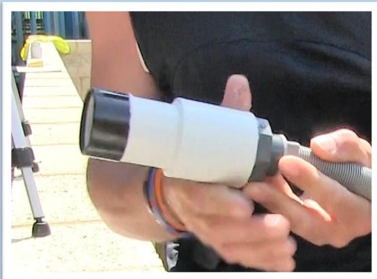
Glue a 50mm slip adaptor on the end of the piece of pipe you have just cut.
