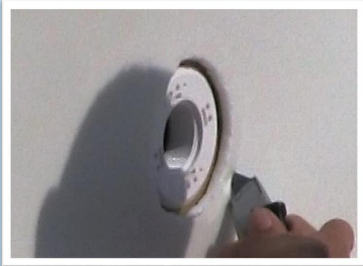
If you have foam on the walls of your pool, you need to cut away approximately 30mm of foam so that the light can be screwed into place nicely without it being too tight against the liner. It is good to cut it with a chamfered edge, to achieve a nice finish when the liner is installed.
