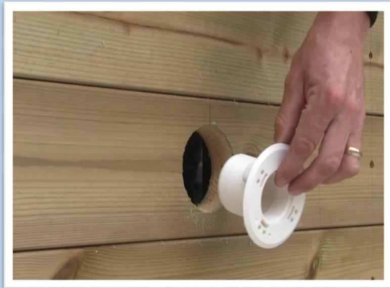
Insert the fitting and tighten against the back nut on the other side of the wall.
