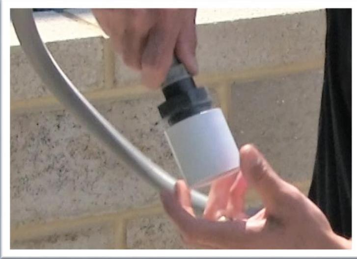
Apply plenty of PTFE to the conduit thread and screw it tightly into the treaded reducer.
