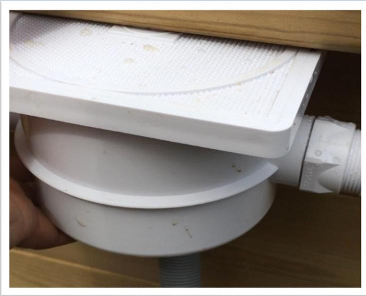
With the other end of the conduit apply plenty of PTFE tape to the thread and screw it into the bottom of the deck box.
