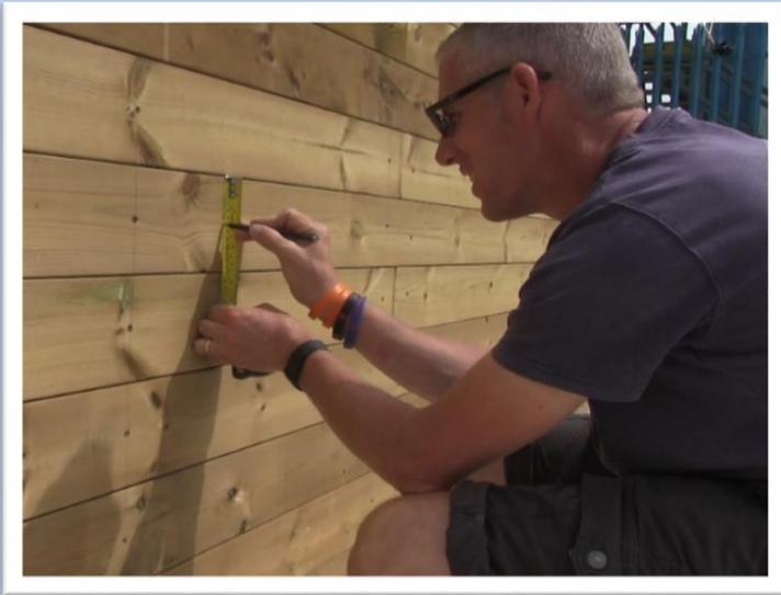
Mark the position where you would like to install a light. Be aware of any vertical supports or other obstructions behind the wall. This is to ensure the back of the light fitting will not foal against anything.
