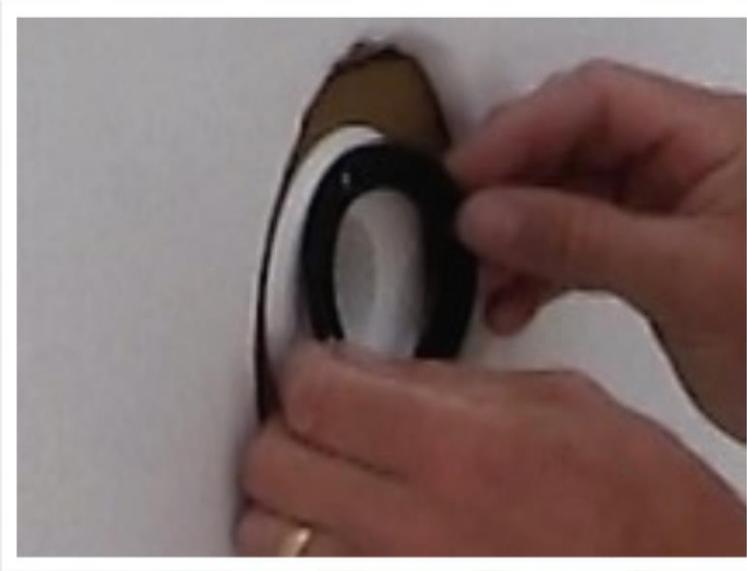
Stick the gasket in place lining up the screw holes.
