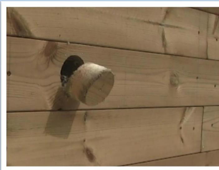
Go around the other side of the wall and drill from both sides to cut a neat hole without any splintering.
