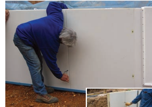
Day 4 - Installing the insulated panels
